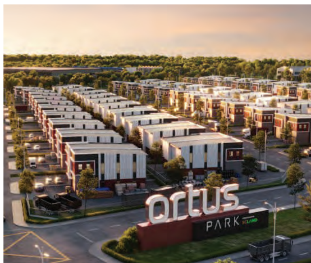
Ortus Avenue, Phase E4 Shop Lot
